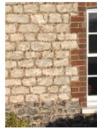
Coursed, galletted chalk with flint plinth
