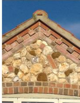
Gable with mortar verges and red brick detailing
