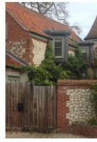
Feature windows finished in grey
