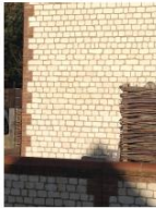
New coursed chalk with brick quoins
