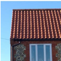
Steep pitched roof with Norfolk red pantiles
