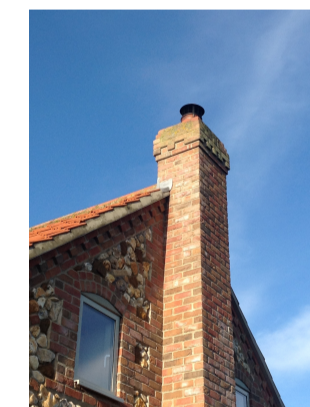
Gable with chimney stack
