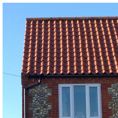
Steep pitched roof with norfolk red pantiles
