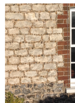
Coursed, galletted chalk with flint plinth
