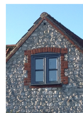
Rough coursed chalk gable
