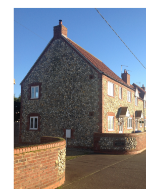
Brick and flint garden walls, characteristic porches and detailed quoins
