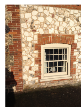
Window with reclaimed brick quoins finished in white
