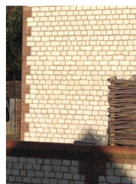
New coursed chalk with brick quoins
